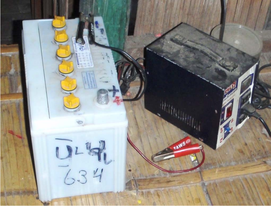
Figure 4: Motor Vehicle Batteries in Camp Homes
