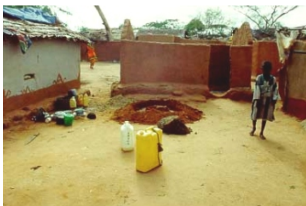
House mudding. Soil, sand, water and manure are used to construct homes.
